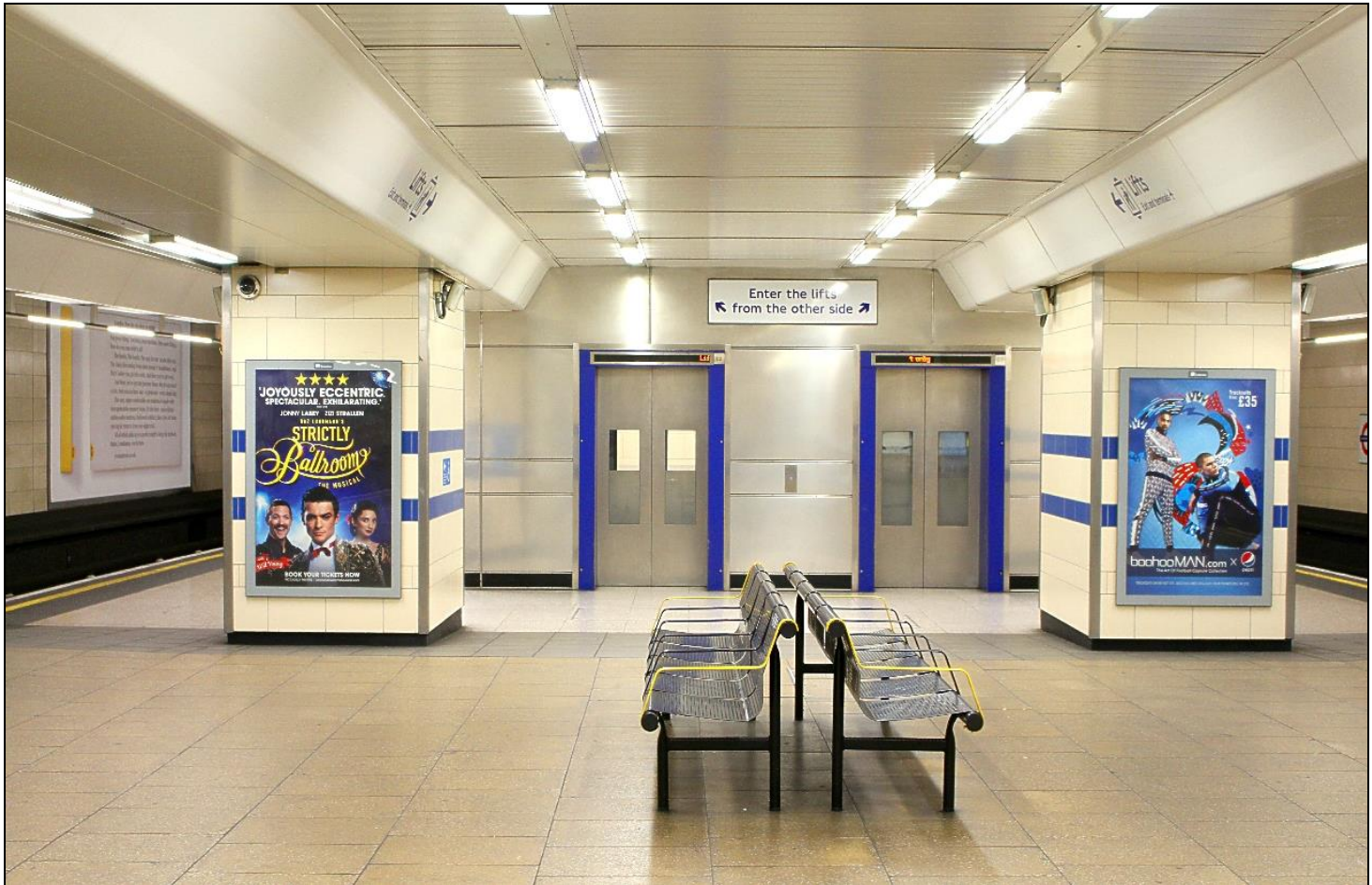
Below: The exit side from the pair of lifts at Heathrow T2,3.
